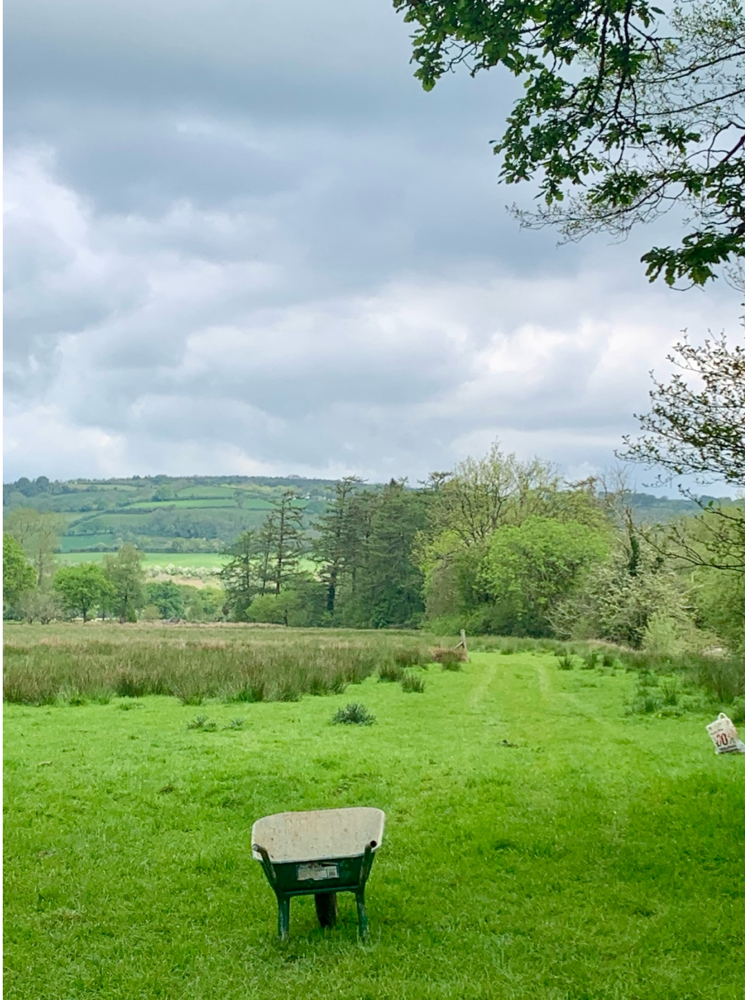
Image 1: Excavation site at Llanllyr facing north (Stewart, 2026 a)
