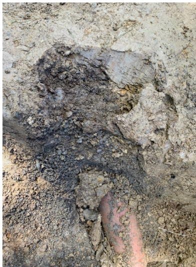
Image 10: Ceramic Land drain with infill on top (Stewart, 2026 i)
