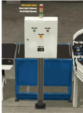
Figure 6 – Control panel and conveyor weigher
