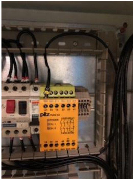
Figure 29 - PILZ Safety Relay
