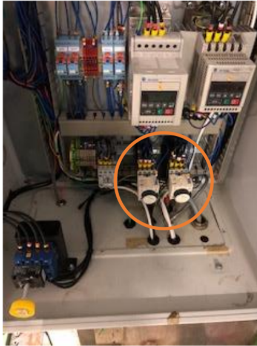
Figure 27 - Contactors with timers
