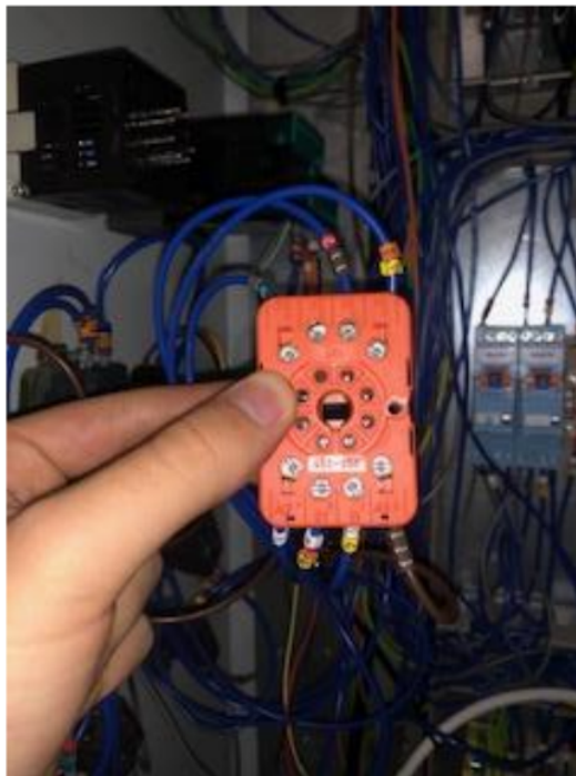
Figure 34 - Timer Connections
