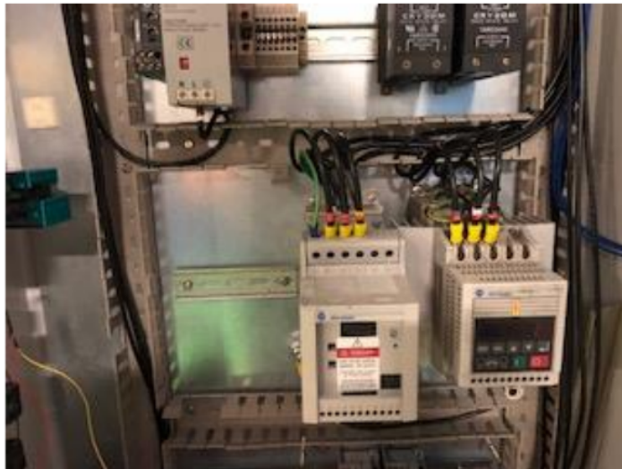
Figure 26 - Inverter Drives
