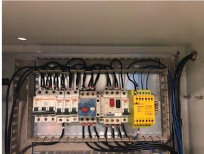
Figure 25 - Wiring the MCBs and Overloads
