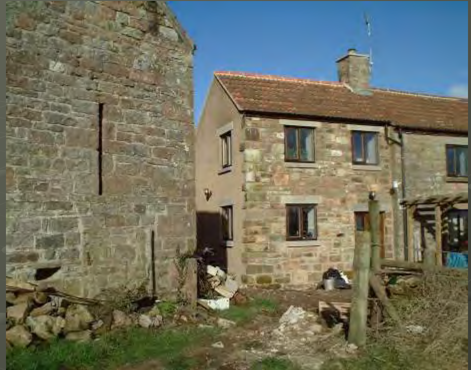
Example of a 17 th century solid wall constructed cottage with 21 st century partial filled cavity wall constructed extension
