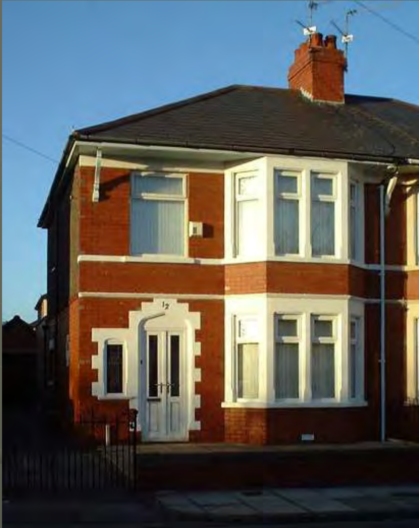
1930's semi detached house with cavity wall construction
