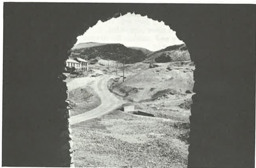
Penrhiw Engine Shaft. Looking towards Bwlchgwyn and Llwynteifi from inside the masonry tunnel, Note the abandoned row of miners' cottages on the left.
