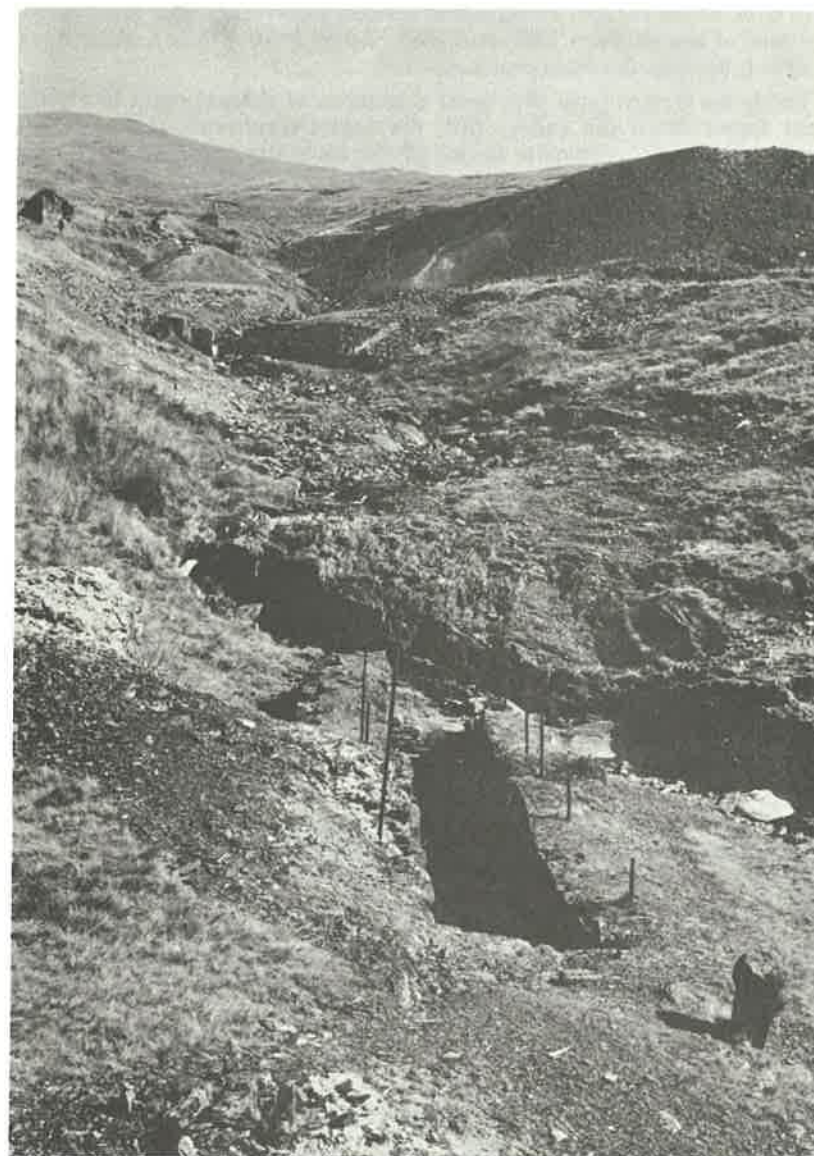
Plynlimmon A view of the mine from the pumping waterwheel pit
