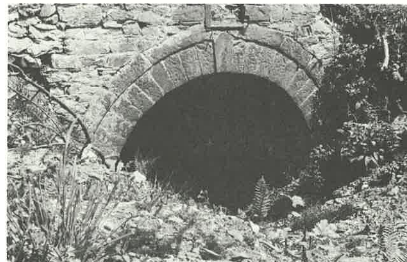
The portal of Taylor's inclined shaft, 1974. Monuments such as this are worthy of protection and restoration.
