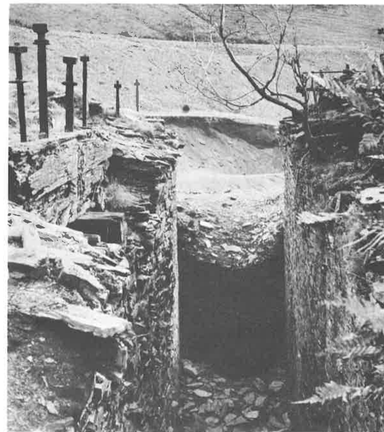
Cwmbwyno. The pit of the waterwheel for driving the crushing machine. Note the massive holding-down studs.
