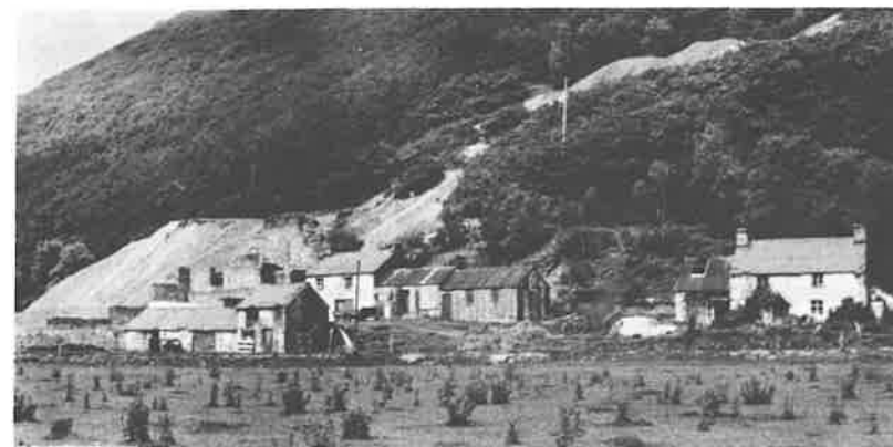
Caegynon. A cluster of mine buildings. Above the dumps at the western end is an old adit, from which a steep path ascends to further adits and the engine shaft.
