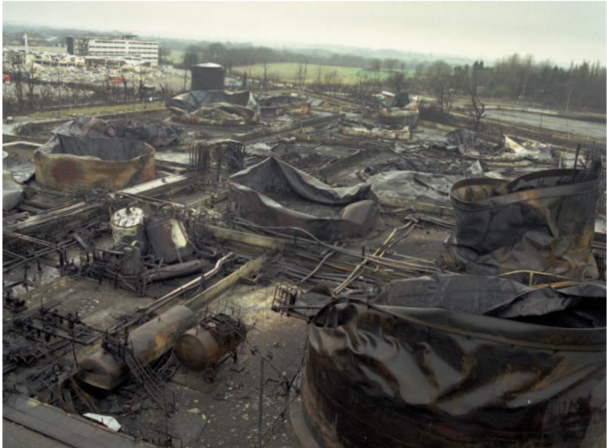
Figure 3: Aftermath of Buncefield Fire (Buncefield Major Incident Investigation Board, 2005)
