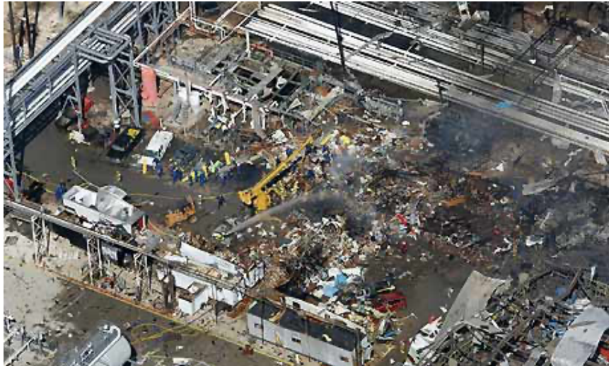
Figure No.2 – Damage after the explosion [4]
