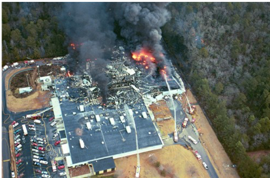
Figure No.3 – Damage after a dust explosion [5]
