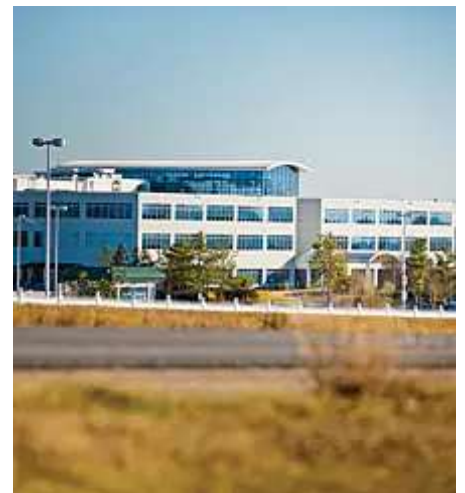
The Hyundai manufacturing plant in Montgomery, Ala., opened in 2005.
