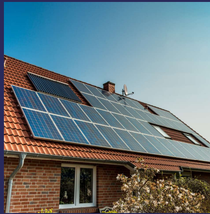
Solar panels on roof (and equipment) Borwick Development Solutions v Clear Water Fisheries [2019] EWHC 2272 (Ch)
