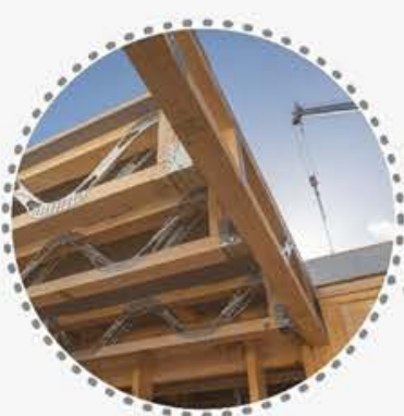
OFFSITE LEVEL 1 SUB - ASSEMBLIES
