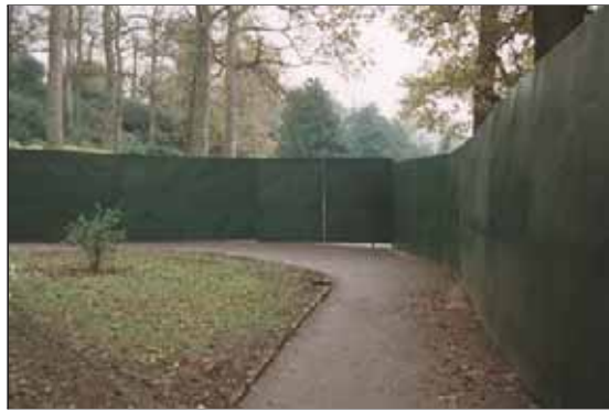
Figure 10.4 Steel panel hoarding
