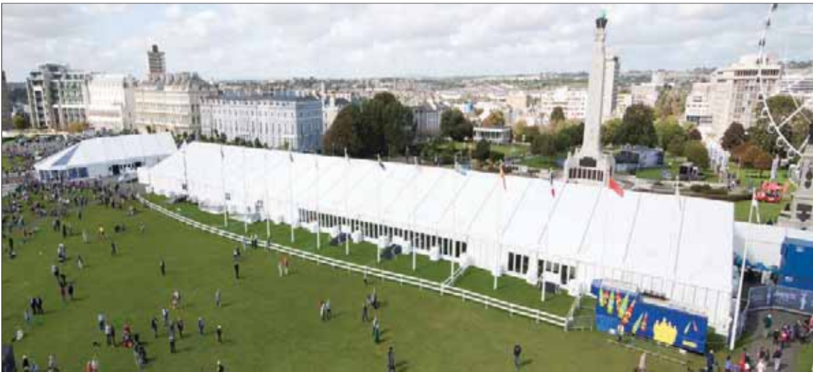
Figure 11.2 Framed fabric structures
