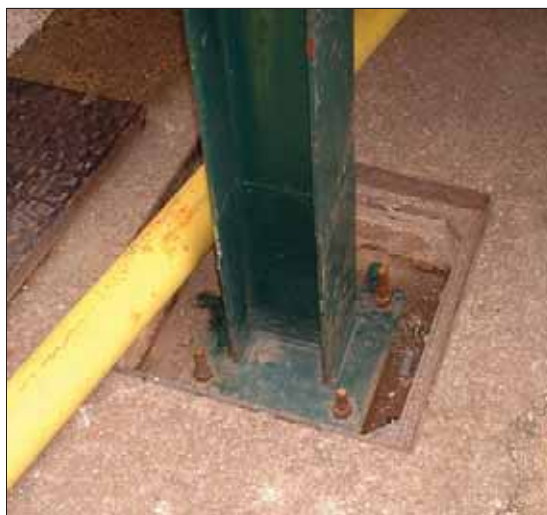
Figure 5.1 Permanent base for frequent re-use
