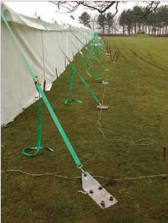
Figure 5.6 Baseplate with four steel stakes
