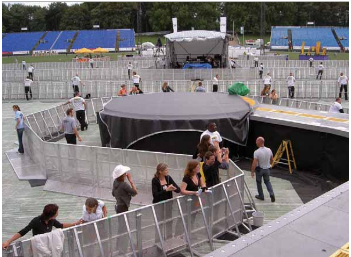
Figure 10.10 Complex multiple barrier arrangement
