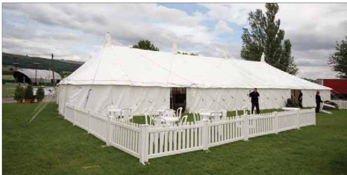
Figure 11.1 Traditional unframed structure
