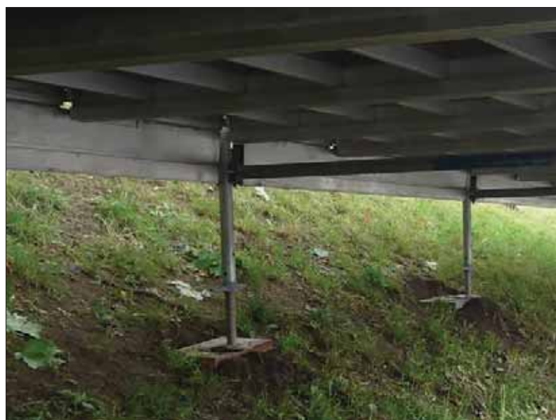
Figure 5.8 Structure on sloping ground
