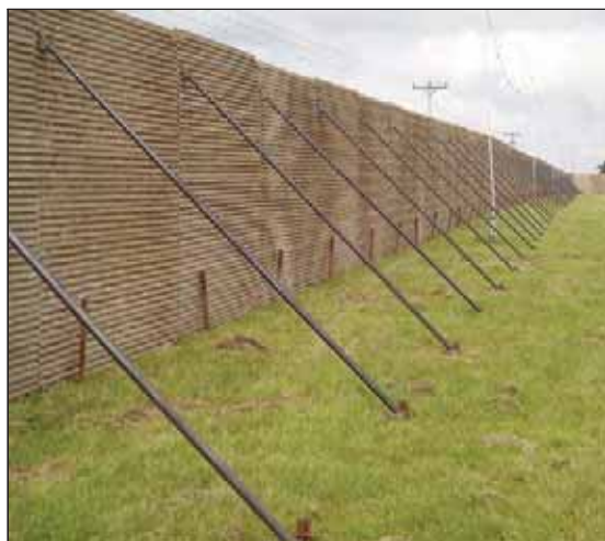
Figure 10.5 Roadway panel system used as barriers/hoarding
