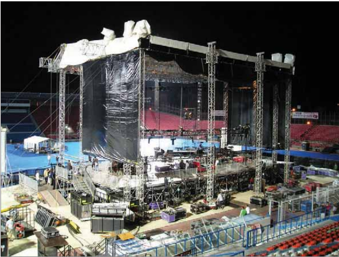
Figure 6.3 Ground support roof structure with large stage structure below
