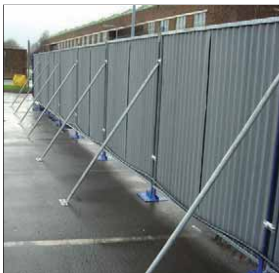
Figure 10.3 Rakers situated between panels
