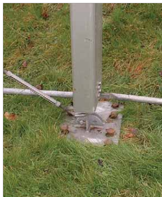
Figure 5.2 Frame marquee baseplate
