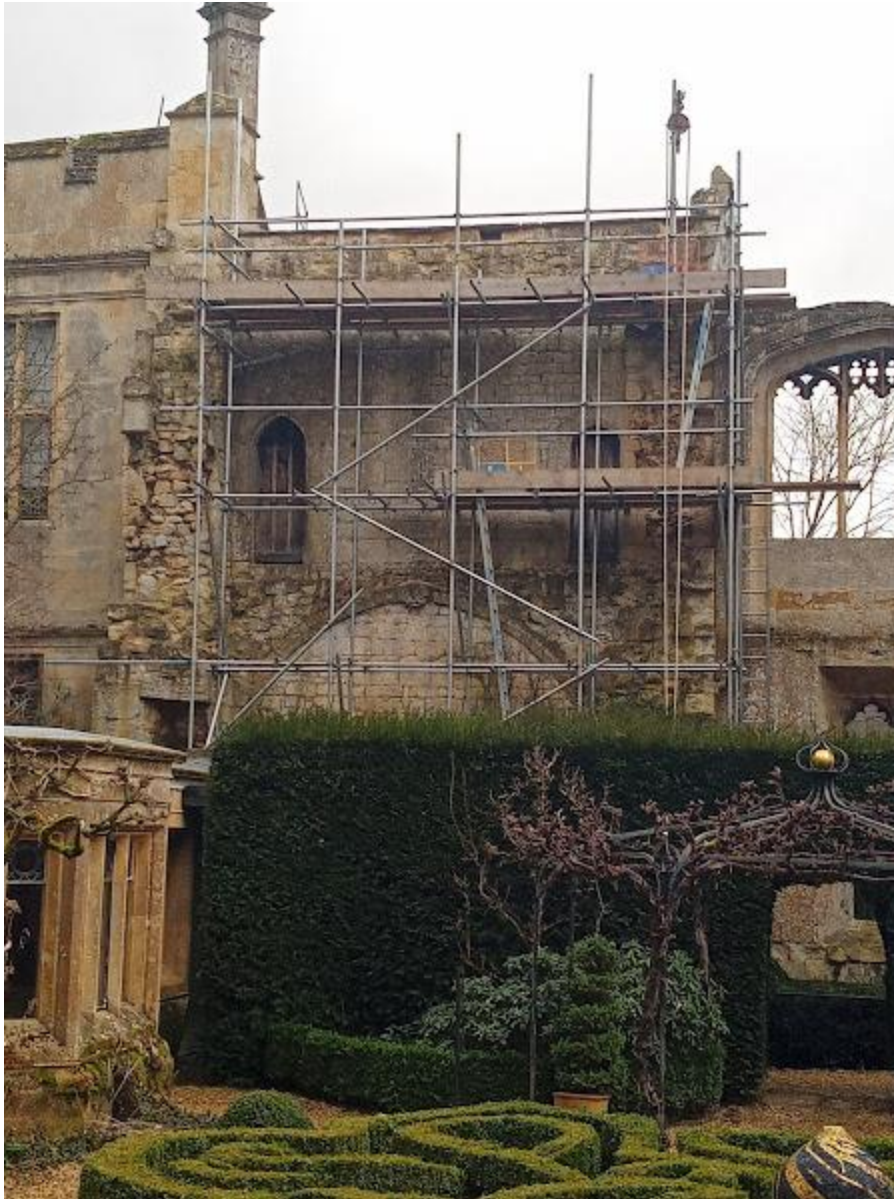
Figure 16: View of medieval arch in missing Cross Range area, 2023
