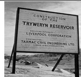
Figure 13 Tryweryn Reservoir Construction
