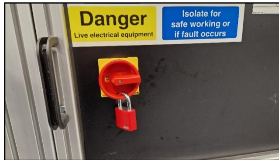
Figure 4 - Power Isolation Procedure
