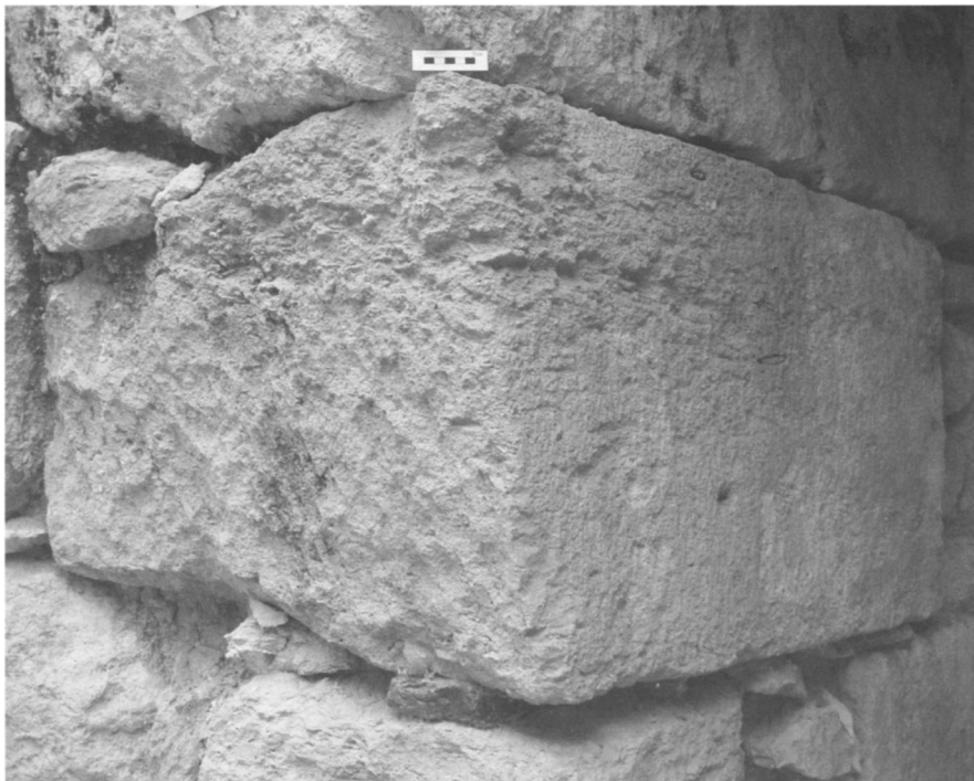
FIG. 8. Comparison of working on the chamber face (to the left) and forehall face (to the right) of the inscribed block.
