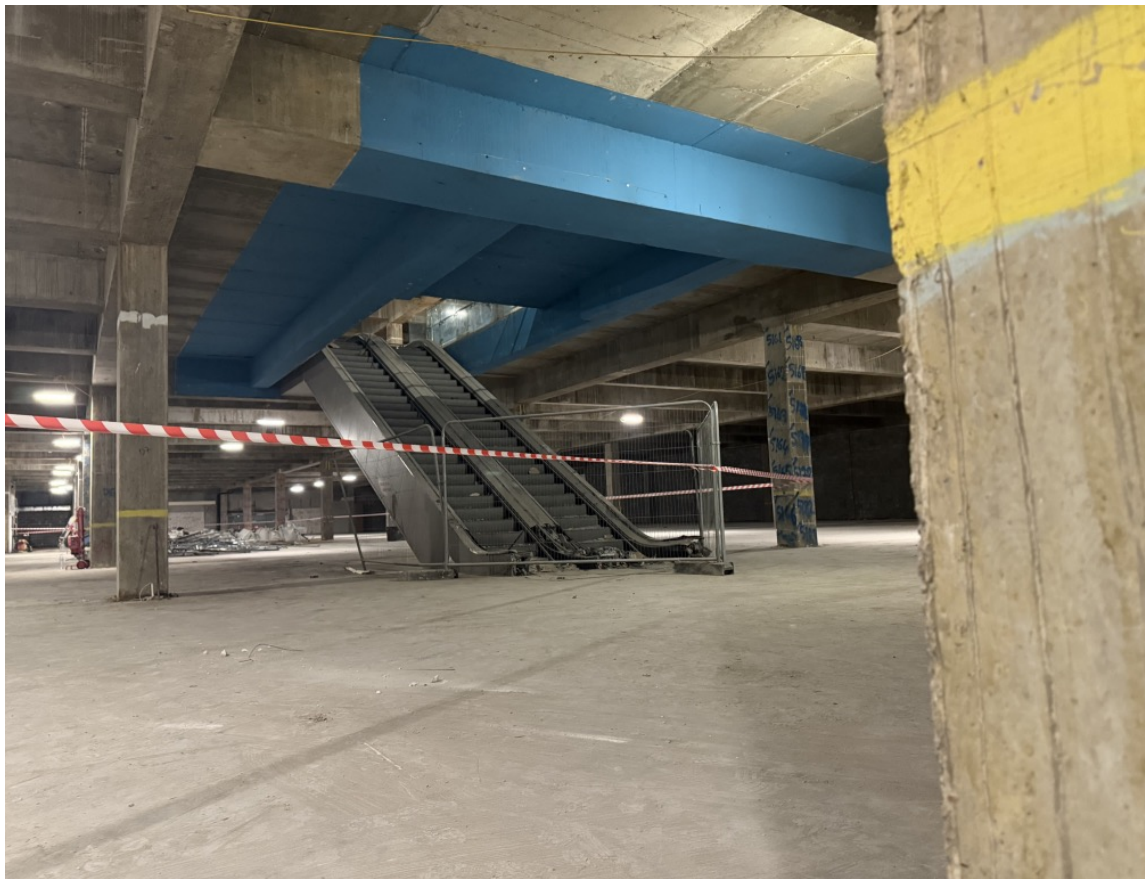
Fig. 7. Abandoned Debenhams Building. (Image: Swansea Council)
