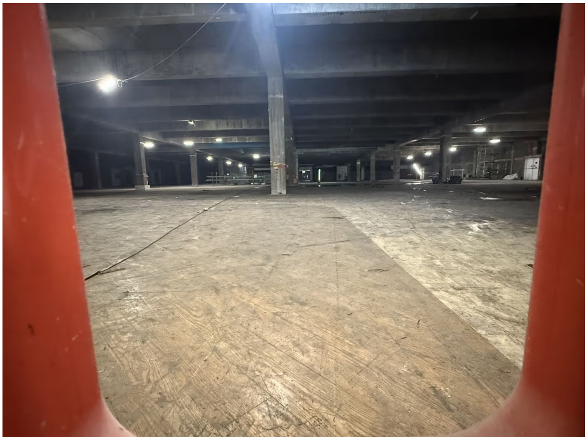
Fig. 8. The Vast Stripped Back Floor Of Debenhams. (Image: Swansea Council)
