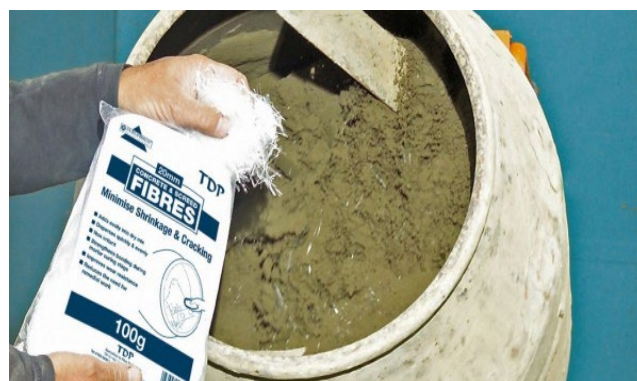
Figure 6: The mixing process of fibres with the concrete mixture.
