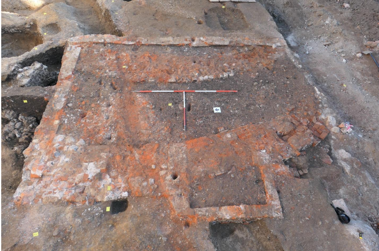
Figure four: A polecam photograph of the brick foundations of the under-stage pit of the Theatre Royal (CAT, 2023).
