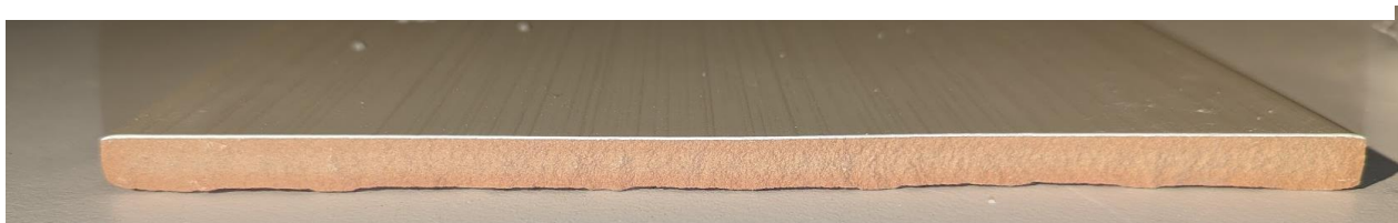
Figure 37 Breaking edge of ceramic wall tile.
