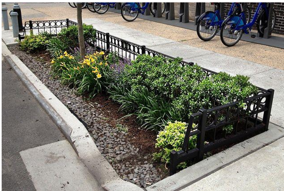
FIG 1. A BIO-SWALE AT 4TH AVENUE AND DEAN STREET IN BROOKLYN. (PHOTO: NYC WATER/Flickr) TAKEN FROM (DWYER, L. 2014).
