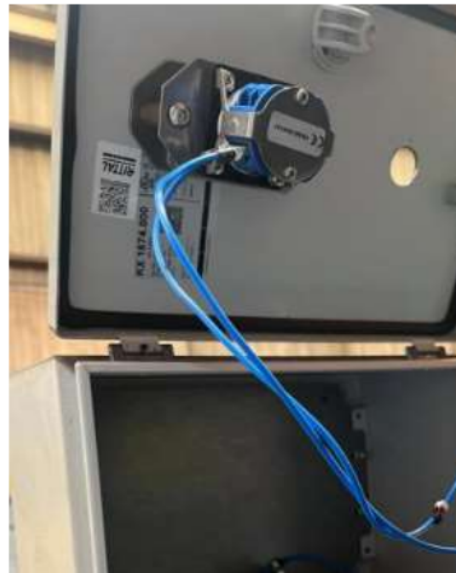
Figure 22 Access key wiring
