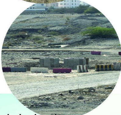
Manhole chambers at the center
