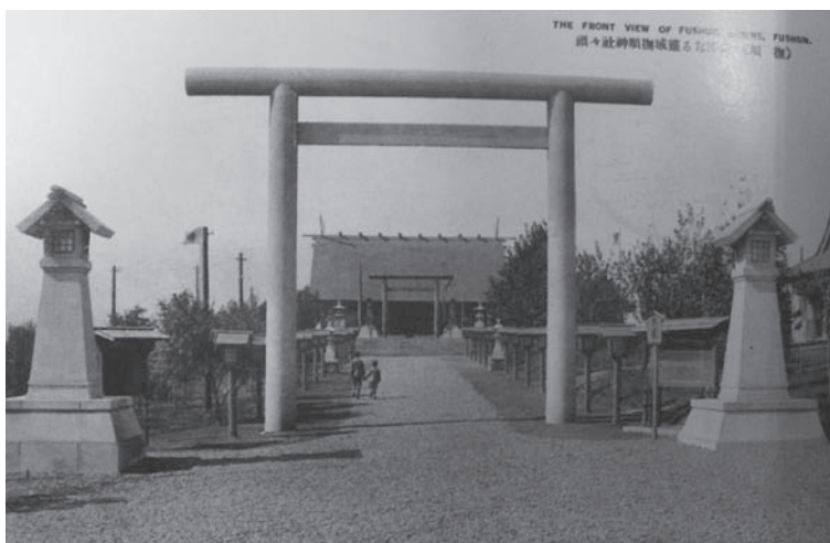
Figure 8.3 Sacred sites in Japanese Manchuria. Shintō shrines were built throughout the empire. Initially for resident Japanese, such shrines were gradually adapted to a program of cultural indoctrination. A. Shintō shrine in the Manchurian city of Xinjing. B. Shintō shrine in the Manchurian city of Fushun.
