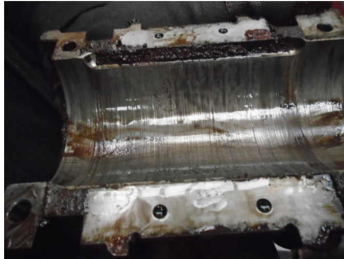
Figure 5 - White Metal Bearing In Poor Condition With Grooves Cut Into The Metal
