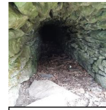
Image 48: Inside the adit (Own Image, 05-05-2025).
