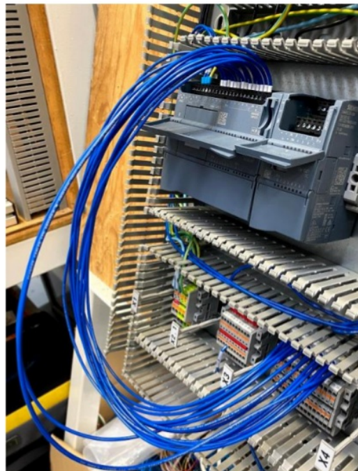
Figure 41 – PLC Inputs to X3 Terminal Block
