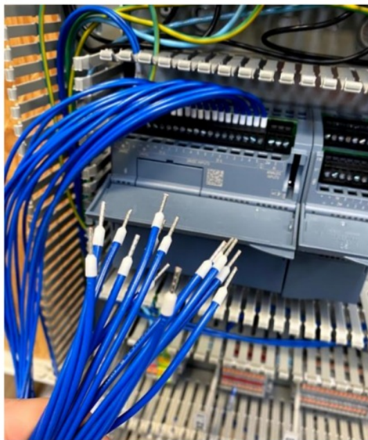
Figure 40 – PLC Wiring
