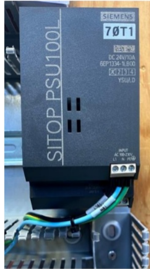
Figure 38 – PSU Wiring
