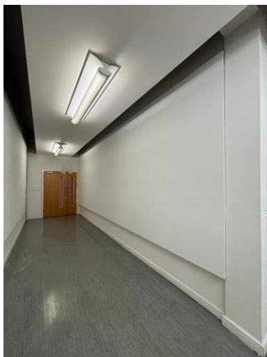
(Initial Corridor Space)
