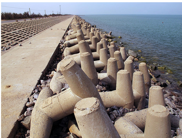
Fig. 3 The 114-km-long shore protection structure defending Gudong oil field on the Yellow River delta
