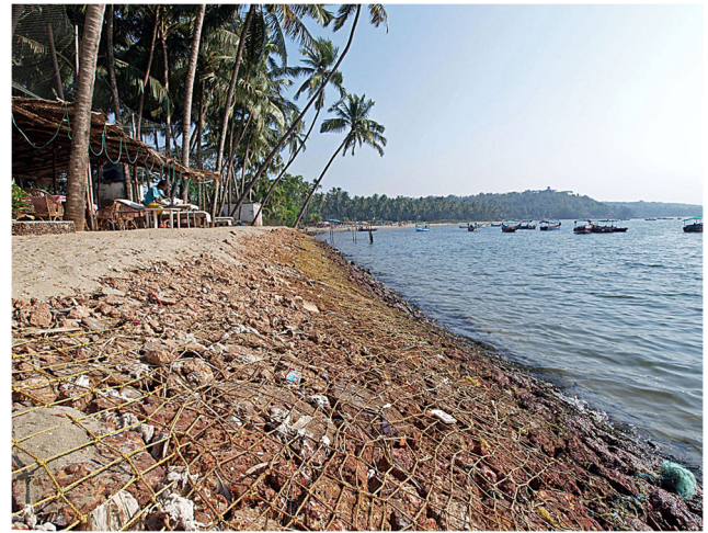
Fig. 4 Rope network holding small stones in a revetment at Coco Beach (Goa, India)
