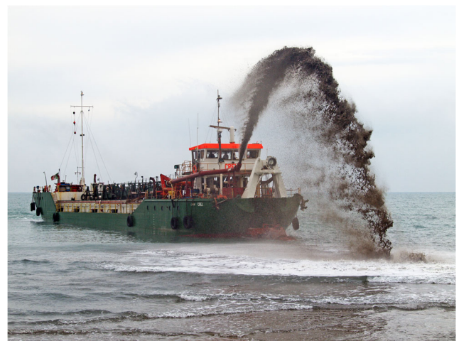
Fig. 5 Nearshore nourishment through “rainbowing” at Grottammare (Marche, Italy)
