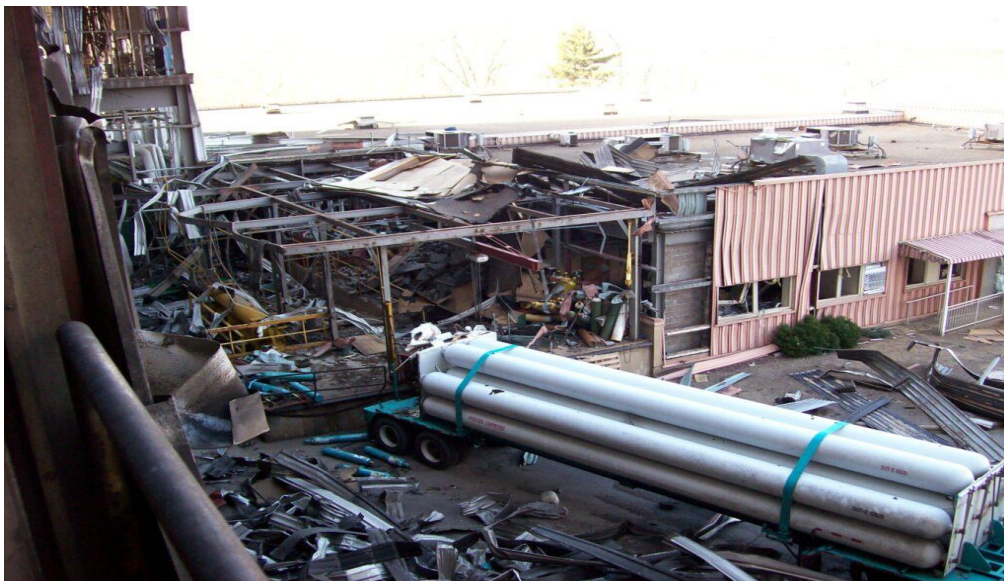
Figure 6: Image showing the aftermath of the Hydrogen explosion (OSHA , 2025).
