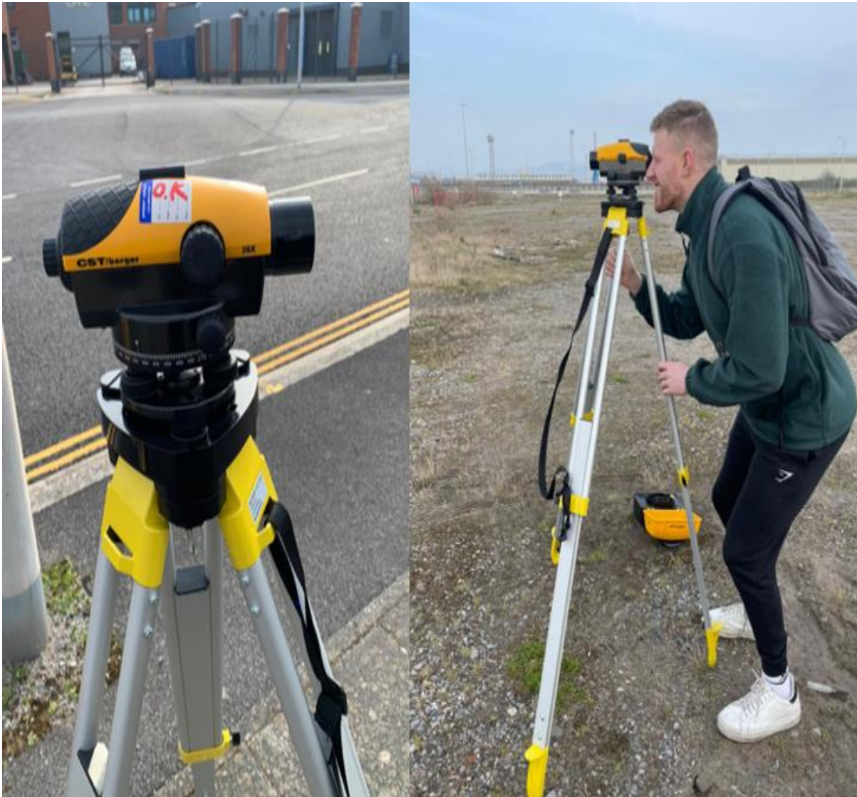
Figure 9: Dumpy level that was used to measure height differences.
