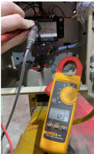
Figure 33 – 12V when PS1 Switched
