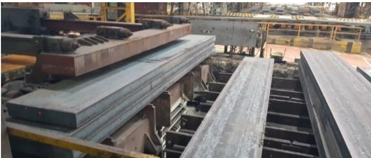
Figure 13 - Magazine used for furnace charging
