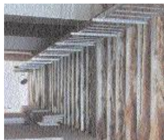
Separating wall using light steel sections
