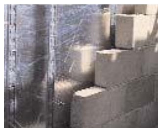
Thermal insulation in an external wall
