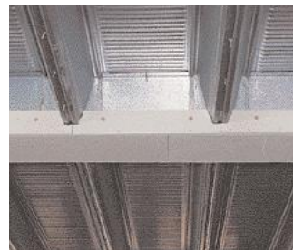
Fire protection to ASB beam
