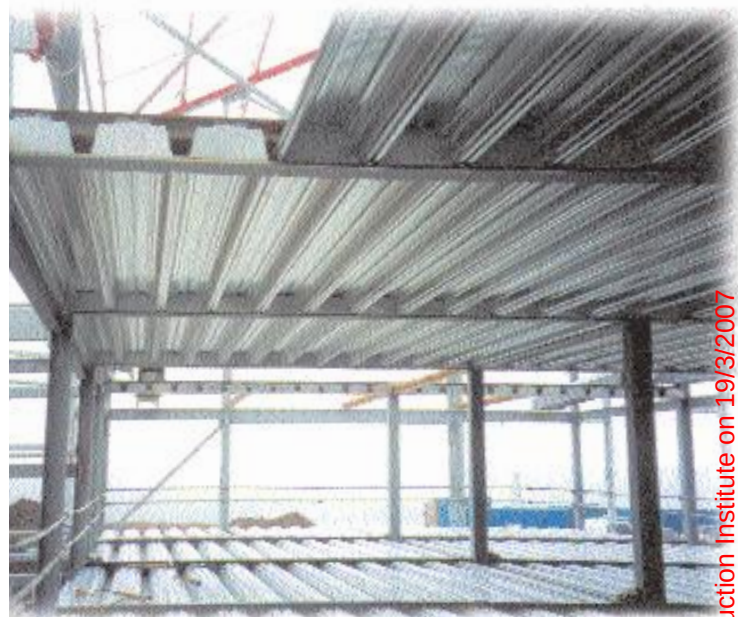
Slimdek ® provides adaptable space by eliminating downstand beams
