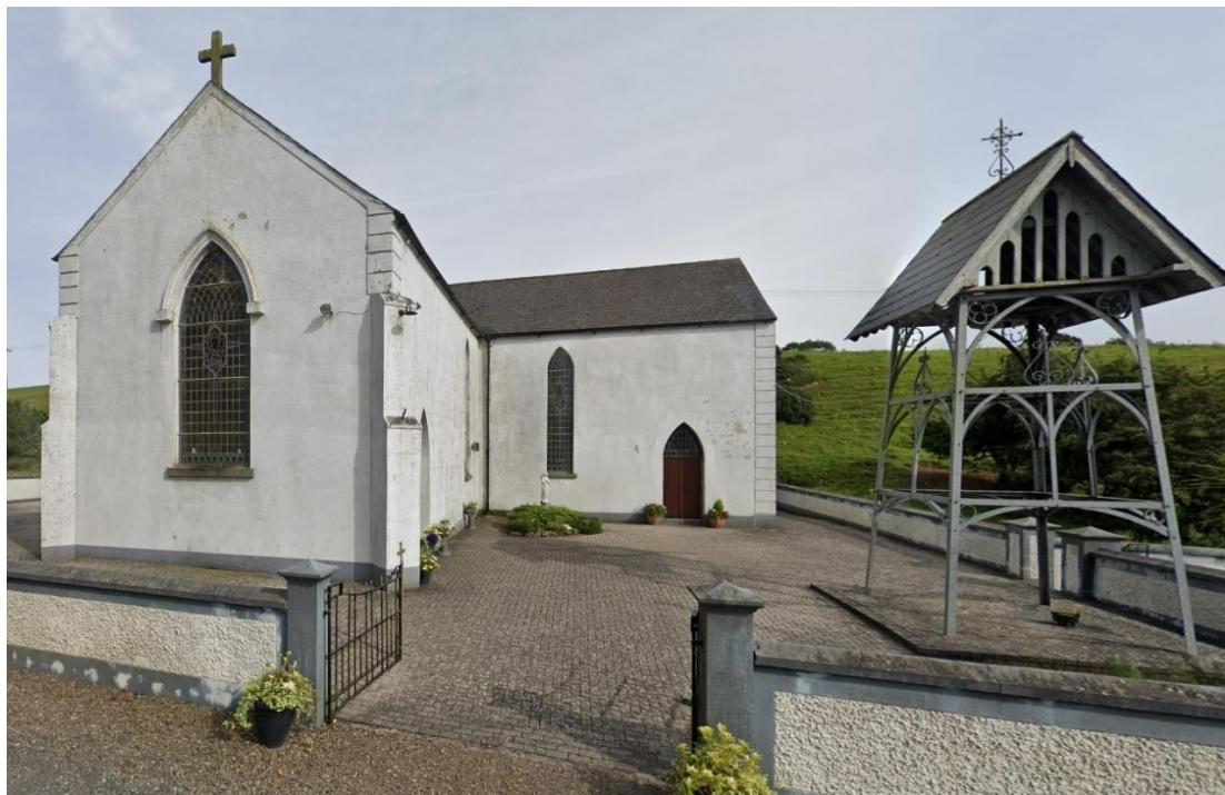
Fig. 7 – The roofed well like structure and apparent well cover outside the Church of St. Brigid Grangegeeth. 232
