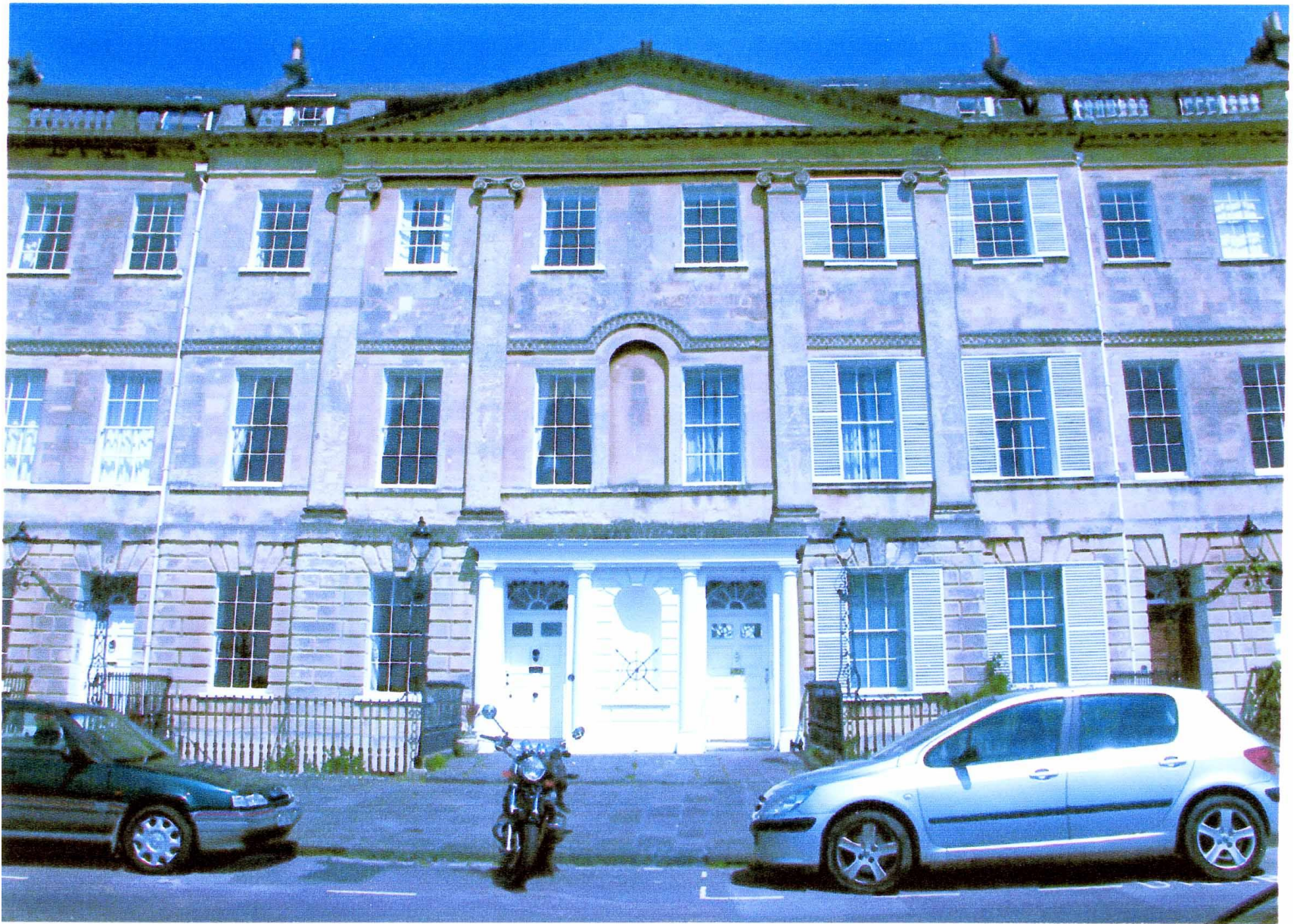
Figs. 12 and 13 Showing the pedimented central feature with Ionic pilasters, and in detail the guilloche scroll over the arched recess.
