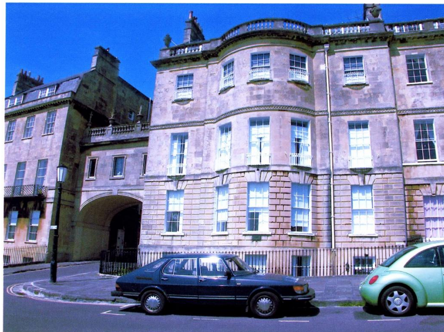
Figs. 14 and 15 Showing No. 20, the western pavilion with a first floor bridge and No. 1, the unbridged east pavilion.
