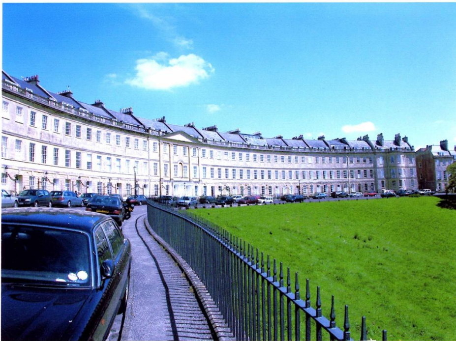
Fig. 11 Views of Lansdown Crescent from the east (above) and west.
