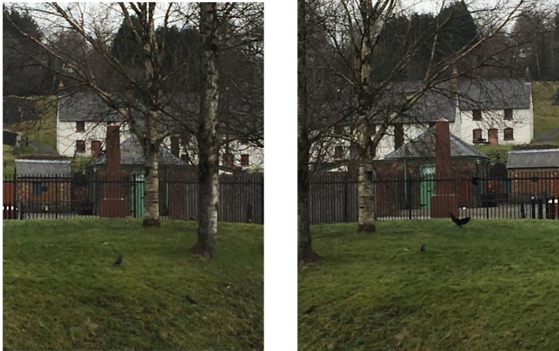
Figure- 3: The Refurbished Stack Square Cottages in the Blaenavon Ironworks yard
