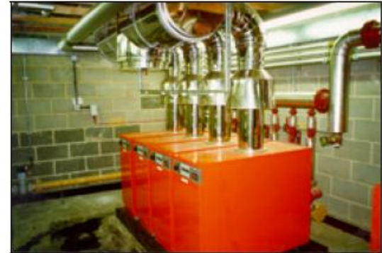
Example of a modular atmospheric gas boiler installation.
