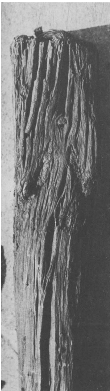
Figure 9. Bruges boat: square form of mast above the two slots which probably contained the halyards (Fig. 7, no. 7; Fig. 23).
