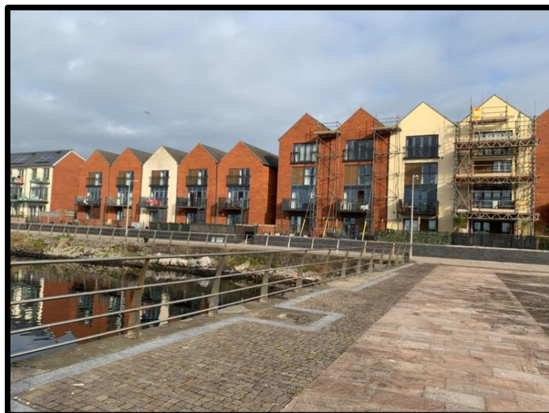
Figure 19: Showing the surrounding developments across the opposite side of the Prince of Wales Dock to our allocated site (Bolton 1902382,2022).
