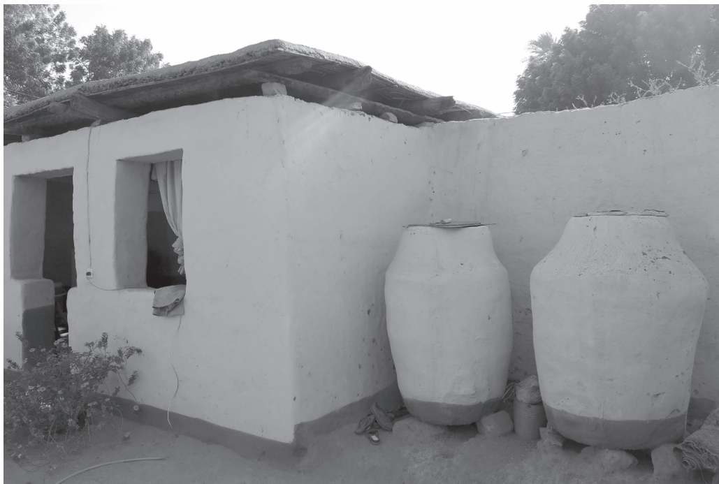
Figure 2.4 Storage bins on Artigasha Island (Copyright, P. Ryan)
