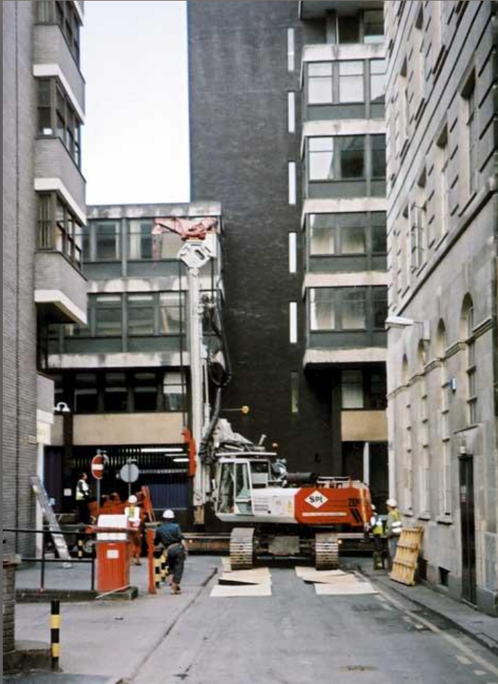
Piling in restricted spaces
