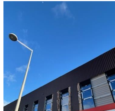
Figure 9 Showing External Building Fabric
