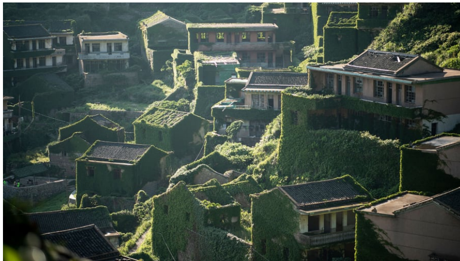
Figure 1 Eisele (N/A) Houtouwan .
