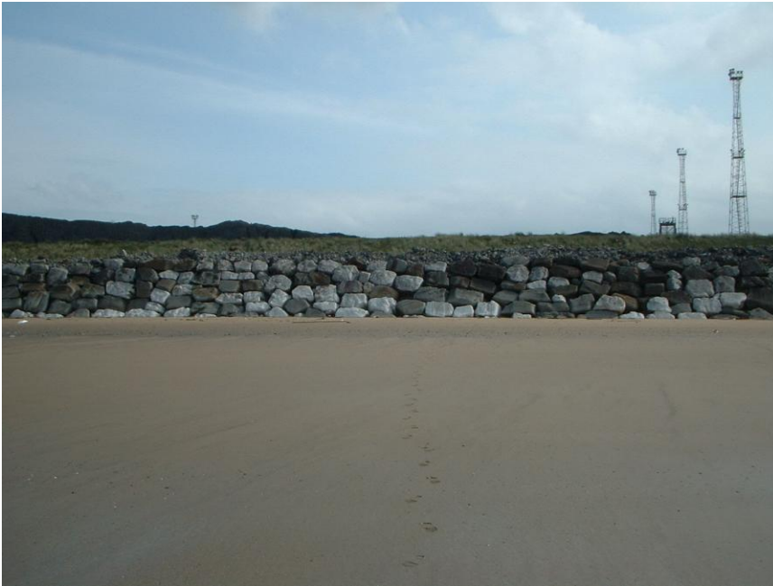
Figure 6: Slag and rock armour revetment (SBCEG, 1999)
