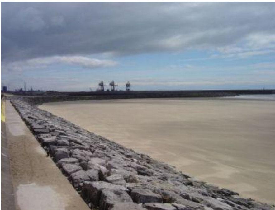
Figure 3: Rock armour fronting promenade seawall
