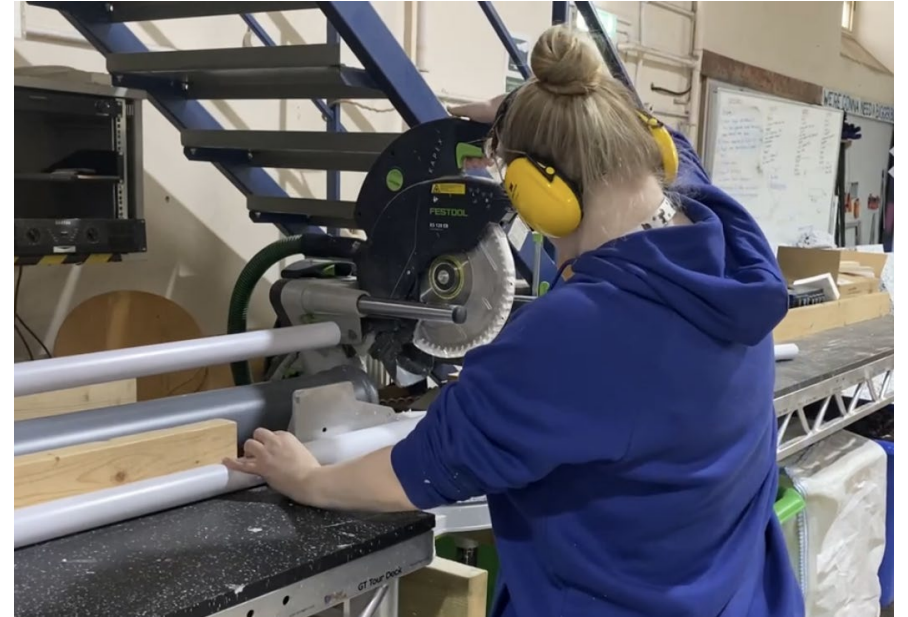
Cutting Pipes to Correct Length
