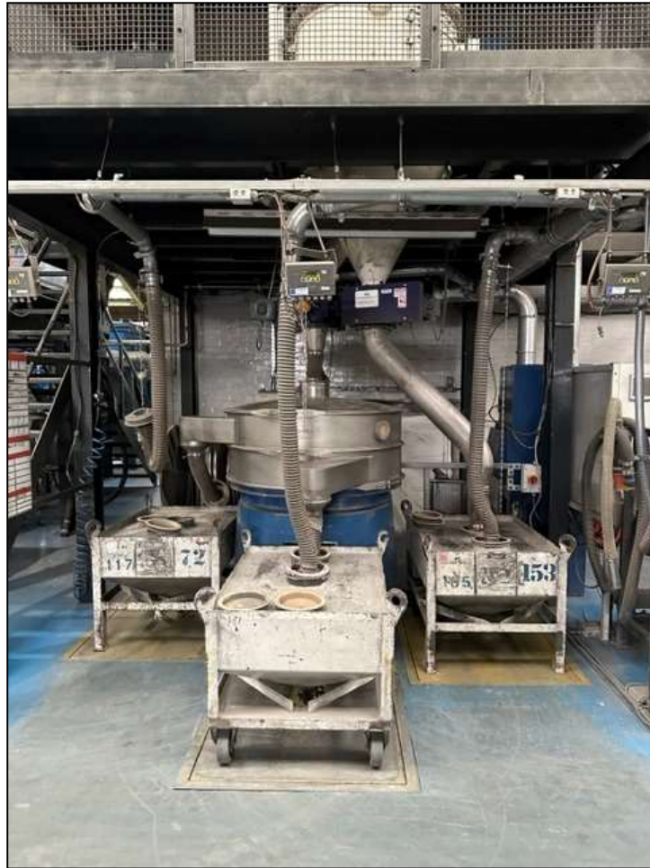
Figure 5 - Vibratory Screening Install at Wall Colmonoy
