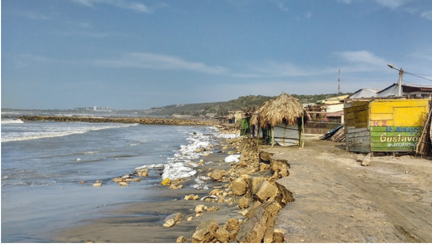
Fig. 7.7 A very low coastal scenic quality influenced by poorly maintained or abandoned coastal protection structures (Salgar, Atlántico, Colombia)
