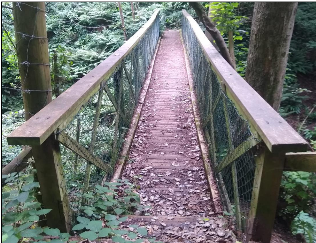
Figure 14. Foot bridge over Holford Glen, July 2023. Photo: Dan Broadbent.
