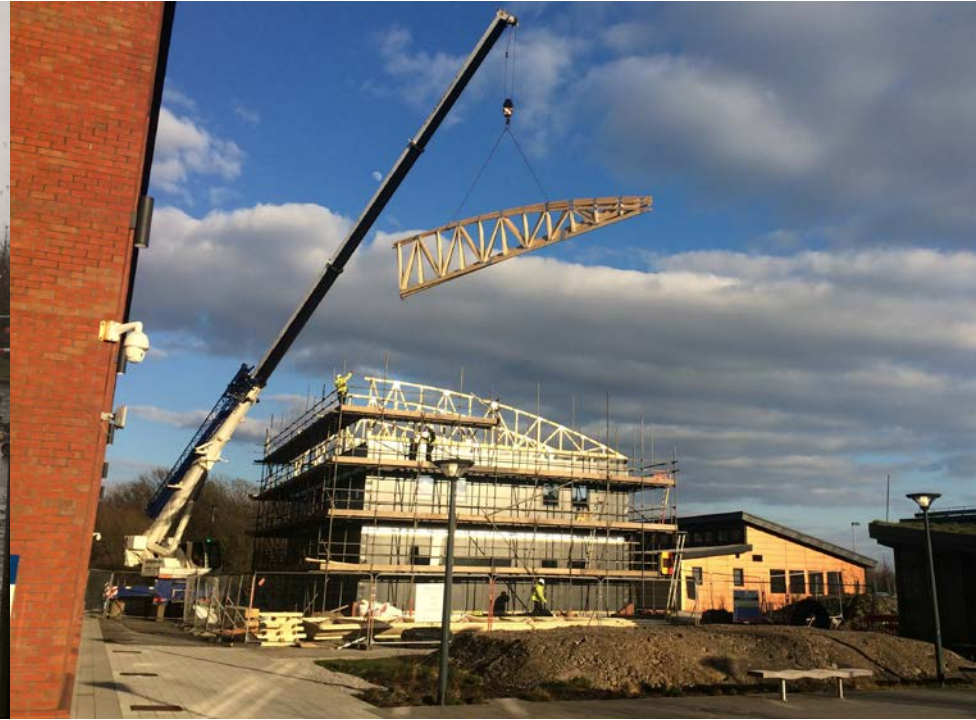
28 th February 2018 – Roof truss installation
