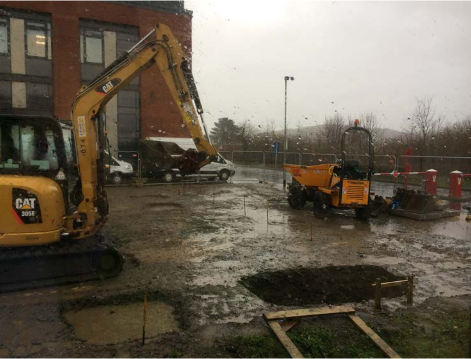
24 th January 2018 - Groundworks
