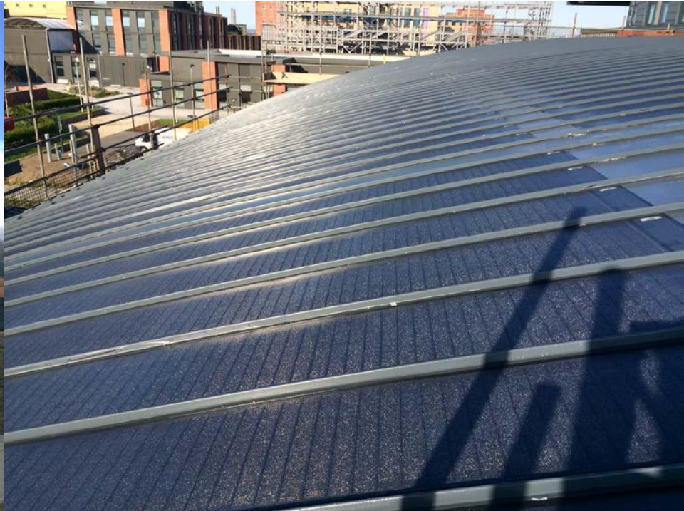
20 th April 2018 – PV Roof complete
