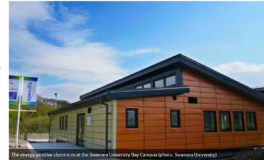
The energy-positive classroom at the Swansea University Bay Campus (photo: Swansea University)
