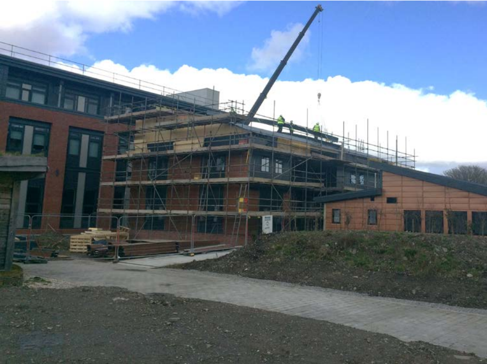
28 th March 2018 – PV Roof Installation
