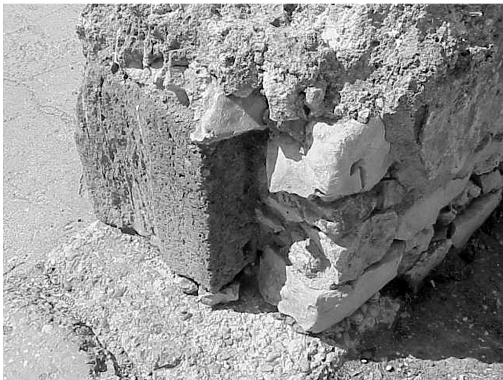
Figure 5.15 Photograph of the east wall of the megaron porch, north of the doorway, showing the presence of reused ashlar blocks, with the dowel hole, originally positioned atop the block, on the interior side of the re-positioned block (photograph by author).
