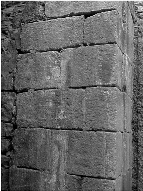
Figure 5.10 Detail of the east stomion of the Tomb of Aigisthos at Mycenae (early LH IIA and LH IIB–IIIA:1), showing the ashlar parastade appended onto the original rubble façade (photograph by author).
