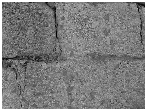
Figure 5.12 (above) Detail of the east stomion of the Lion Tomb at Mycenae (LH IIA–B), showing traces of plaster in the interstices between the blocks (photograph by author).
