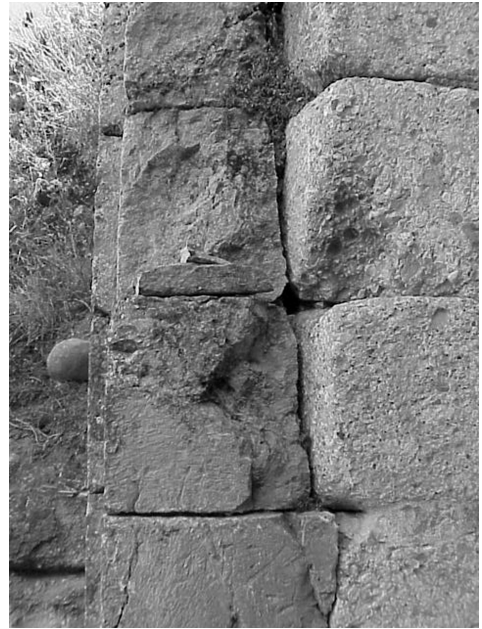
Figure 5.11 Detail of the east stomion of the Lion Tomb at Mycenae (LH IIA–B), showing the ashlar parastade appended onto the original façade (photograph by author).
